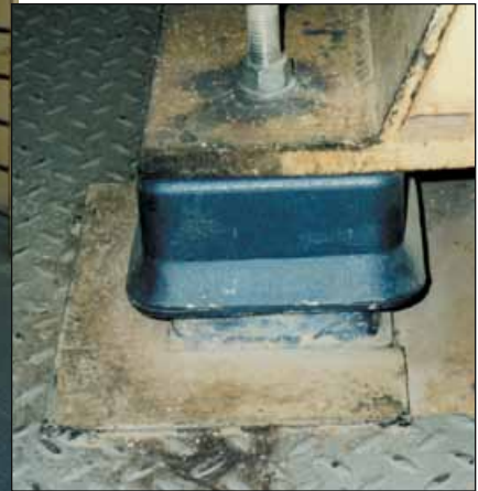
Figure 16 Detail of anti-vibration mount
