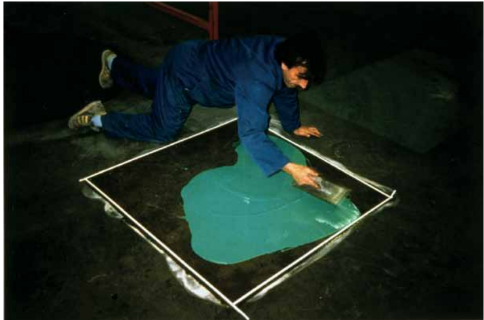
Figure 14 Damping compound being applied to metal decking
