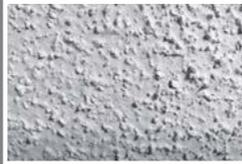
Asbestos textured coating on a ceiling
