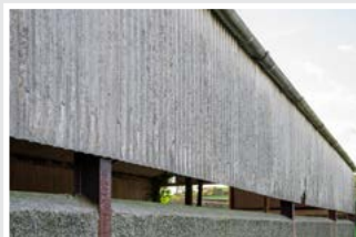
Asbestos cement as fabric of building
