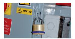
**Step 3** Shut off the power at the main power isolator.
